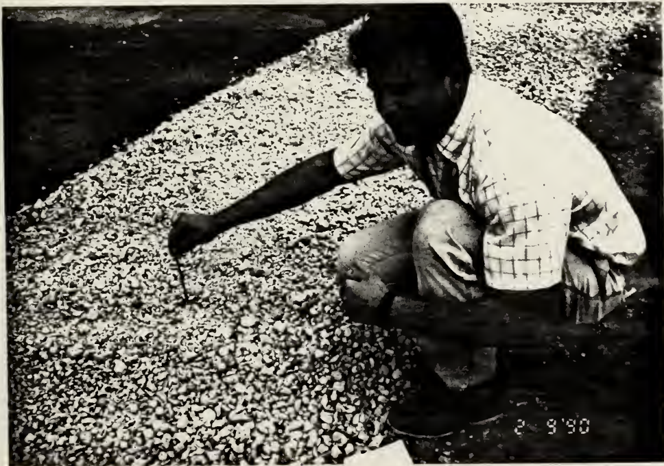
Figure 2.6 Measuring Coarse Aggregate Layer
